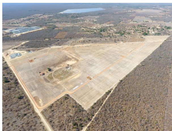
BJL4 Solar under construction (PC: Biosar)
